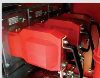
They are provided with single primary winding and single or double secondary winding, depending on the required use.
