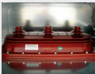
The on-load switches IM6 type, with resin envelop, are filled with hexafluoride (SF6) as dielectric insulation and interruption. Its position creates a separation between the bus bars compartment and the main equipment compartment.
